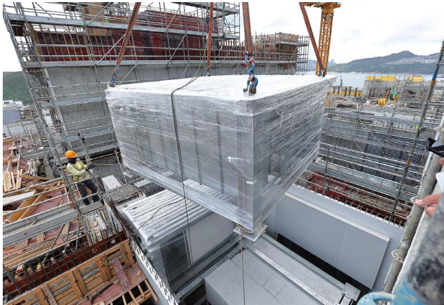
An MiMEP plant room is lifted into position.
